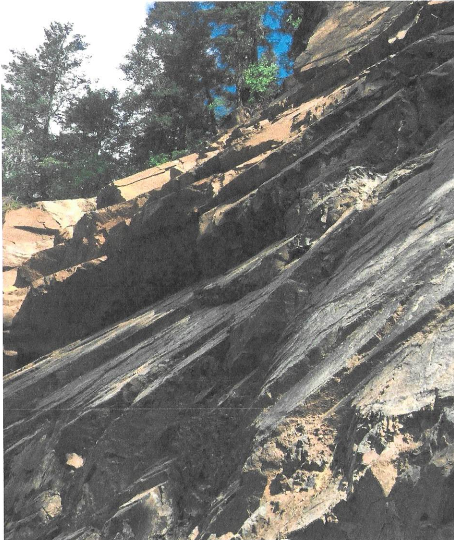
Photo 4. Close up of rock slope, showing dip coincident with the slope.
