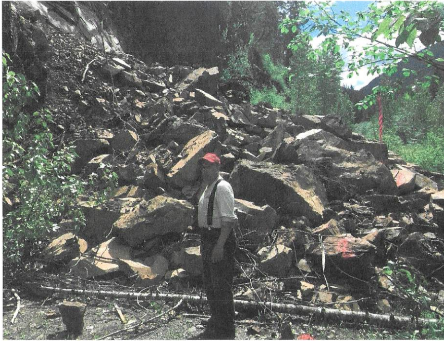
Photo 1. Rock slide deposit has buried the road for an estimated 30 m section
